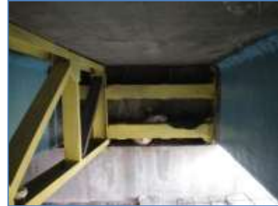
Connection of truss over main beam
