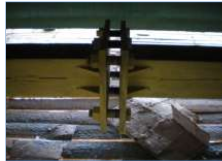
Pre-stressing Mechanism in Truss
