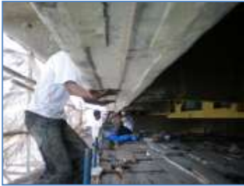
Groove for carbon Fibre composites laminates
