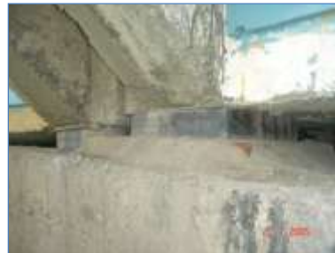
Replacement of damaged Bearings with new
