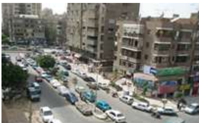
Fig. (28), Nasr City district, buildings have the same style. (Source: Authors)
