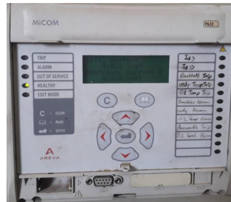
Figure.5 Differential Relay using for Thanlyin Substation
