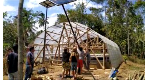
Figure 6. PLTS Installation (2 days)
