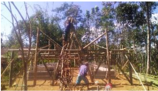
Figure 4. Construction of a Greenhouse (15 days)
