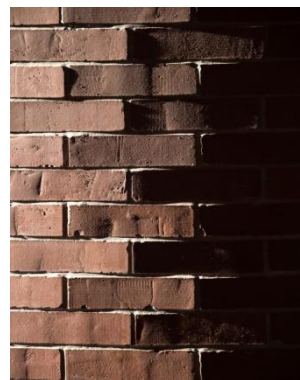
Figure 11. Use of Local Materials
