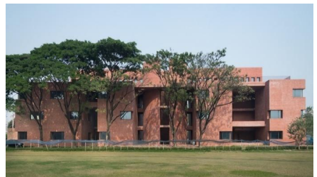
Figure. 7 Front View of Building 1, ULAB
