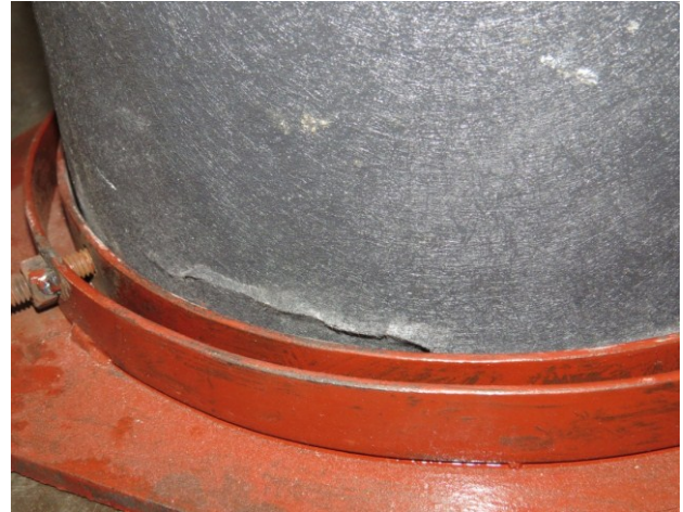
Figure 5 . Crushed at the bottom
