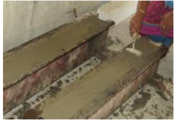
Fig.4 Casting of specimens
